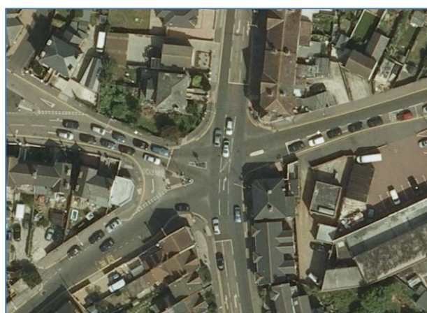
Figure 18 – Victoria Traffic Signals
