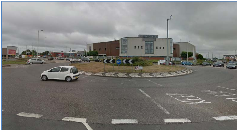
Figure 4 - Westwood Roundabout (A256 / A254)
